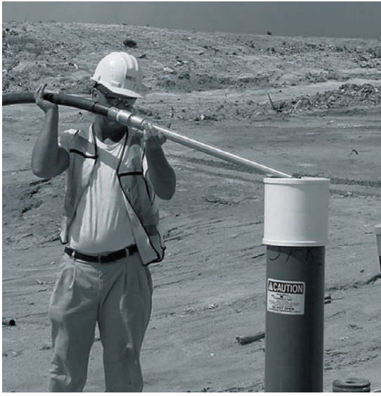
Feed downhole assembly, foot-valve first, into well casing.
