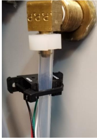
Figure 5-9: Optic sensor tubing installation
