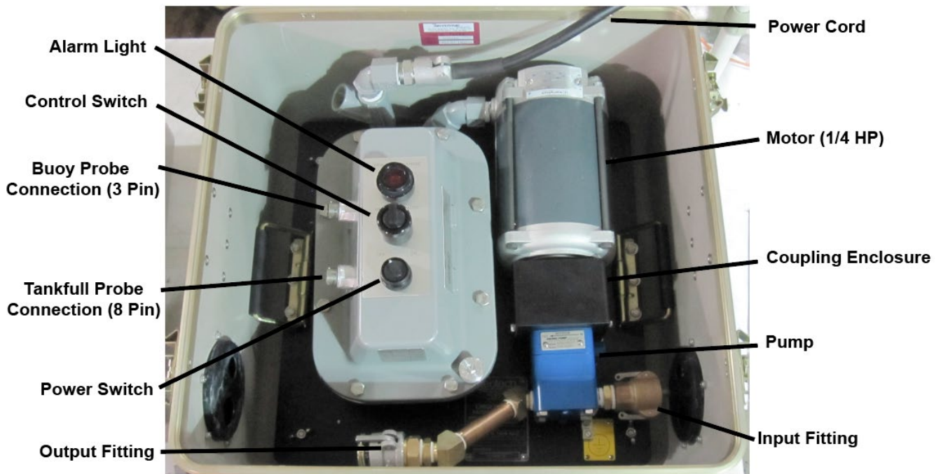
Figure 1-4: New LDFS Pump Control Module Assembly
