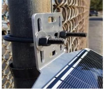
**Figure 2-2:** Fastened Panel with U-bolt
