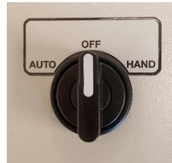
**Figure 3-1:** Example of a HAND/OFF/AUTO (HOA) Switch
